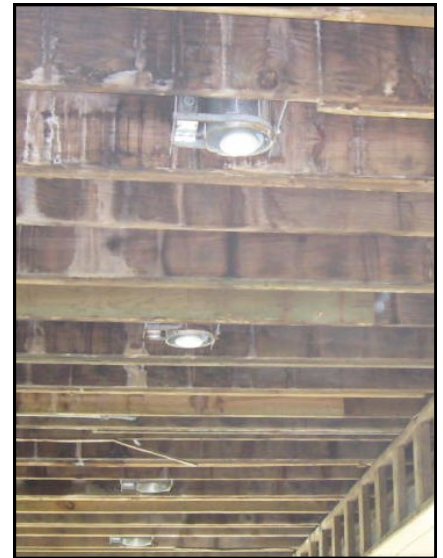
Failed Tile Job
